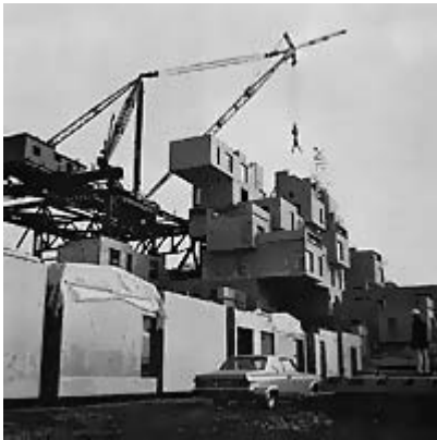
Habitat '67 under construction Bâtiment , June 1967
