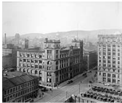
The Grand Trunk and Canadian Express headquarters building, in 1924 Canadian National Railways Headquarters building, McGill College Ave., Montreal, Quebec, c. 1924 , photographer: unknown. Canadian National collection, No. CN000667, Canadian Museum of Science and Technology
