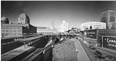
The CN complex under construction, in 1946 Montreal's Central Station, looking north , Montreal, Quebec, 1946, photographer unknown. Canadian National collection, No. CN000148, Canadian Museum of Science and Technology
